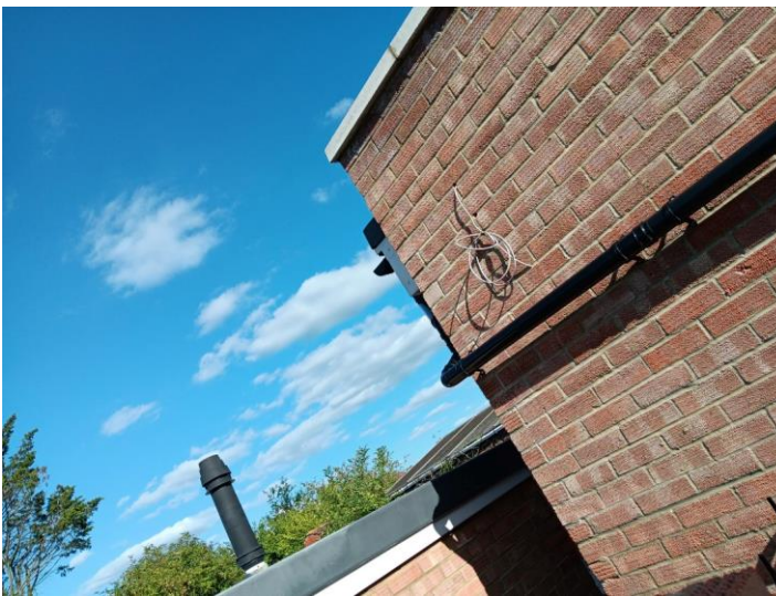
Figure 4 Adjacent property extension and host site existing rear projection/swimming pool
