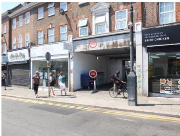
Undercroft approach between 229 and 233 Station Road
